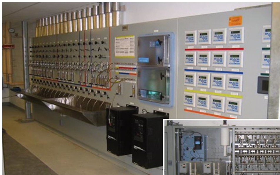
1, 2. Sample panels are among the last items considered in the design of a powerplant and among the lowest in priority for capital upgrades
